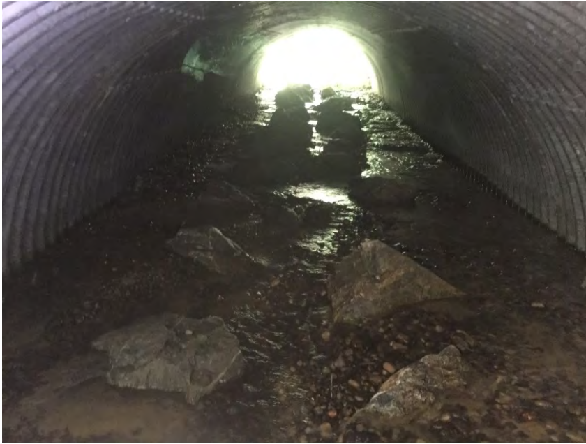
Looking through culvert from outlet
